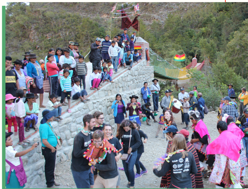
The inauguration day after completing the construction of a footbridge in Chavarrias, Bolivia involved dancing, speeches, and confetti.
